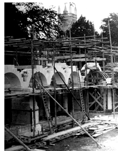
War Cloister under construction.
