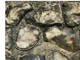
Flint: Wykeham's original building material. Flint for War Cloister was similarly sourced from Shawford.
