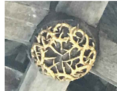
Roof boss of crown of thorns.
